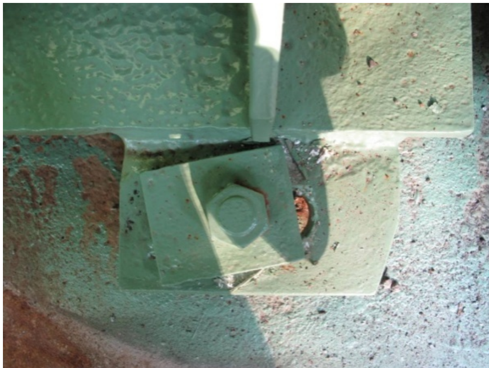
Figure 5-4 Courthouse Road over South Anna River - bearing displacement (37.98064, -78.04818).
